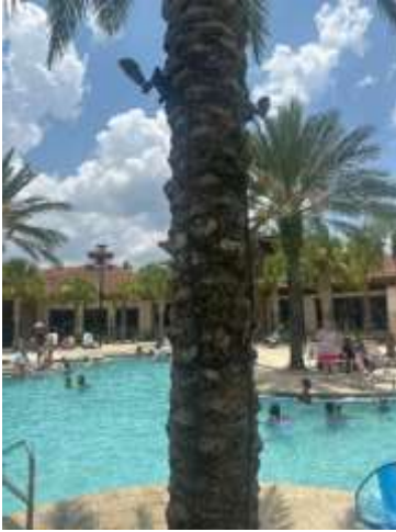
Main Pool Deck Palm Lighting After
